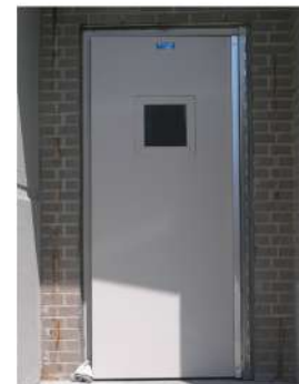
Flood Mitigated Walk Door
