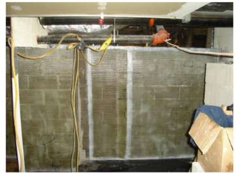
Strengthening Infilled Wall With Composites
