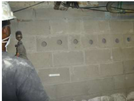
Infilling CMU Wall
